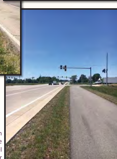
Example Bike Path with Minimum Separation and Bike Friendly Shoulder between Travel Lane and Curb and Gutter
