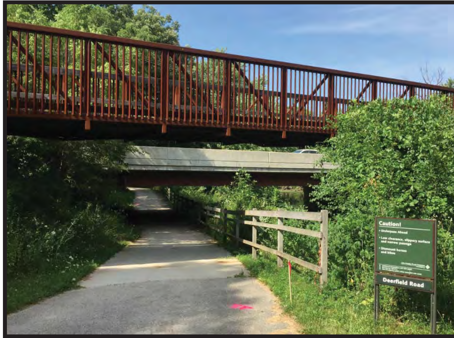
Figure 1-11: DPRT Underpass at Deerfield Road Looking North
