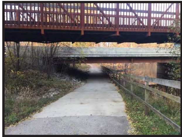
Figure 3-14: DPRT looking north at the Deerfield Road crossing
